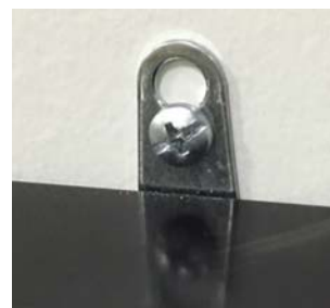
Top mounting shown in photo above with the seismic clip secured to the wall.
